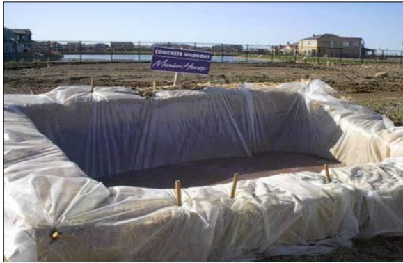
Plate 3-1 Concrete washout area
