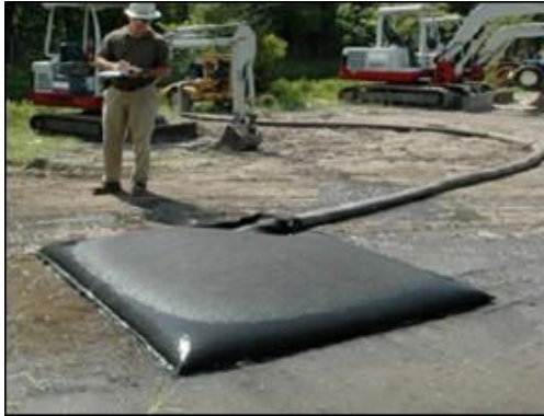
Plate 2-1 Silt Bag with water being pumped through
